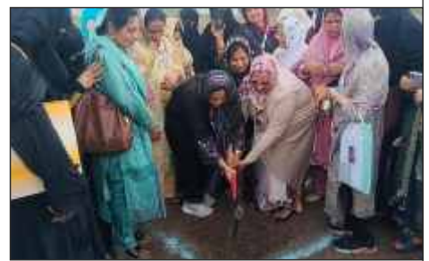
Mrs. Asfiya Afzal Padela & Mrs Naseema Surty breaking the ground with a spade for the foundation stone laying ceremony of AIMJF Degree College
