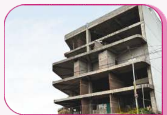
NEW UNIT UPCOMING IN BILASPUR
